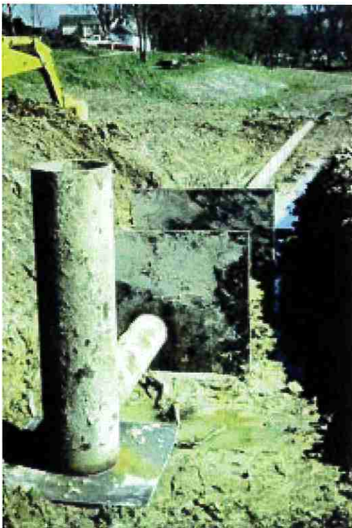
Figure 22 Drop-inlet pipe spillway with antiseep collar
