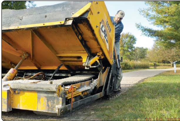
Resurfacing the stone trail beside the barn.
