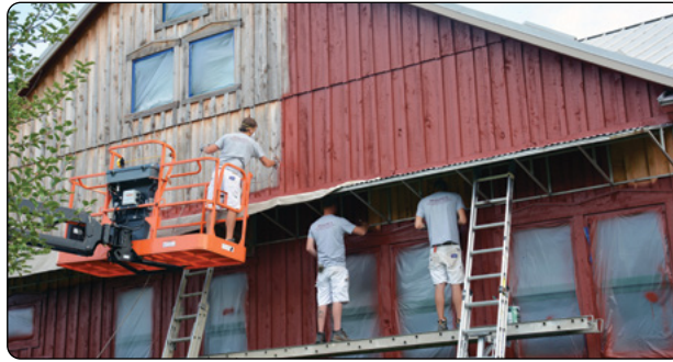
Applying red stain to the new hemlock barn siding.
