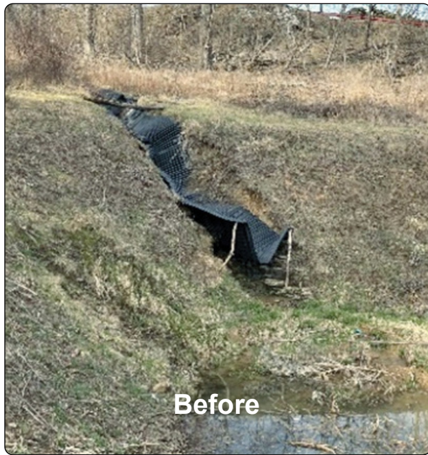
Dilapidated plastic channel (left) replaced with riprap channel (right).
