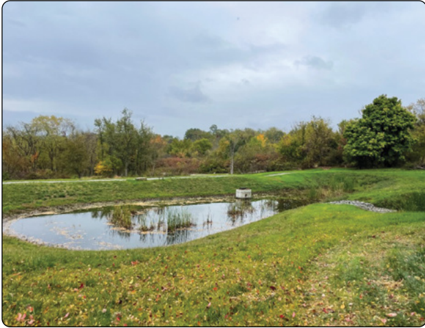
The completed basin with a trail along the embankment.
