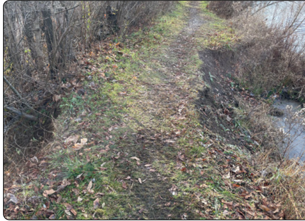
Saint Vincent Lake's embankment parallels Fourmile Run and has been eroding, compromising the lake's integrity.
