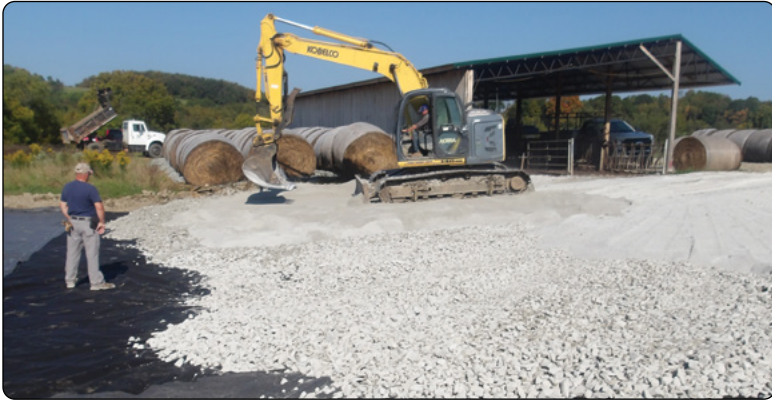
Contractor installing the stabilized AHUA.
