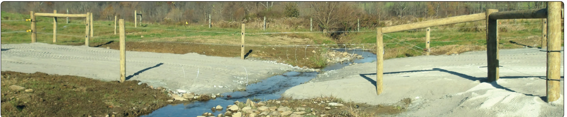
A stabilized stream crossing installed that allows cattle to cross and access drinking water.
