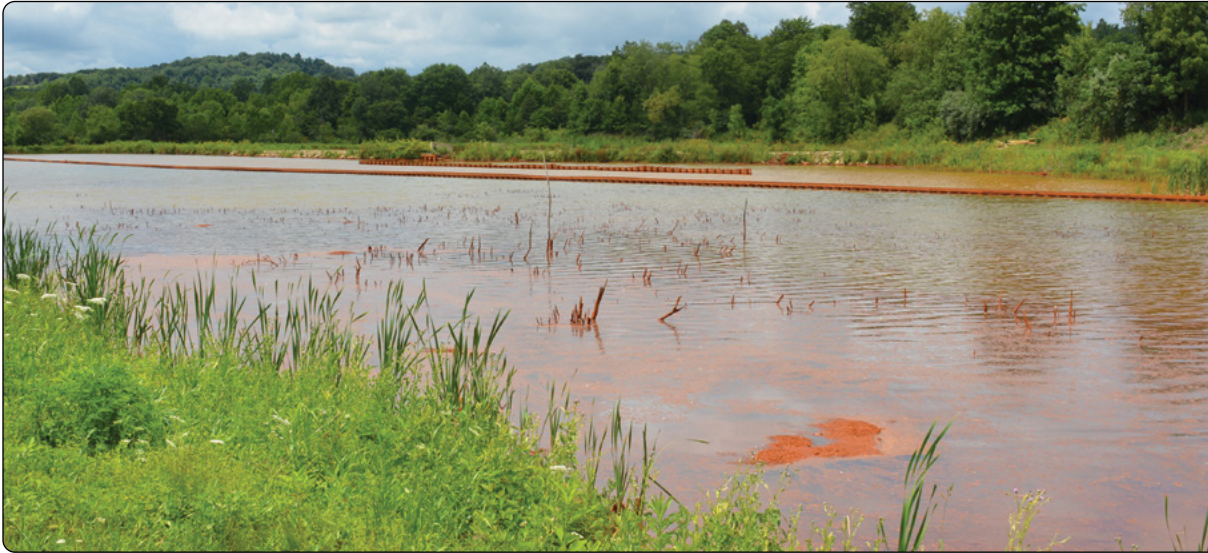
Baffles at the Brinkerton site (the dark orange linear objects in the treatment pond towards the top of this photo) help direct discharged mine water through the treatment system. This helps iron oxide pollutants to settle out.
