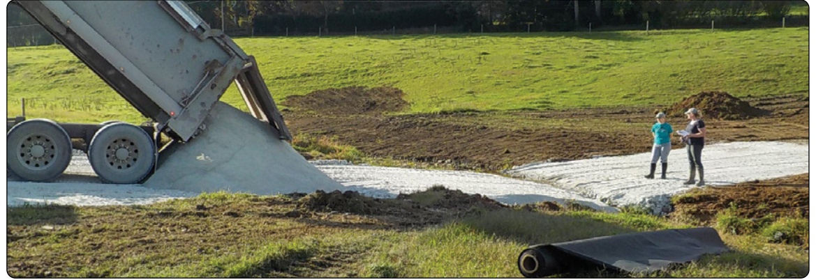
WCD staff ensuring the stabilized stream crossing is installed properly.
