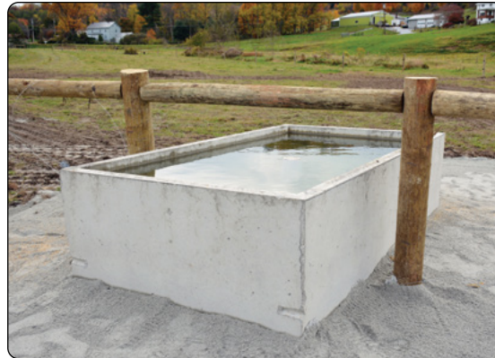
Spring development with a watering trough between the stabilized AHUA and pasture.
