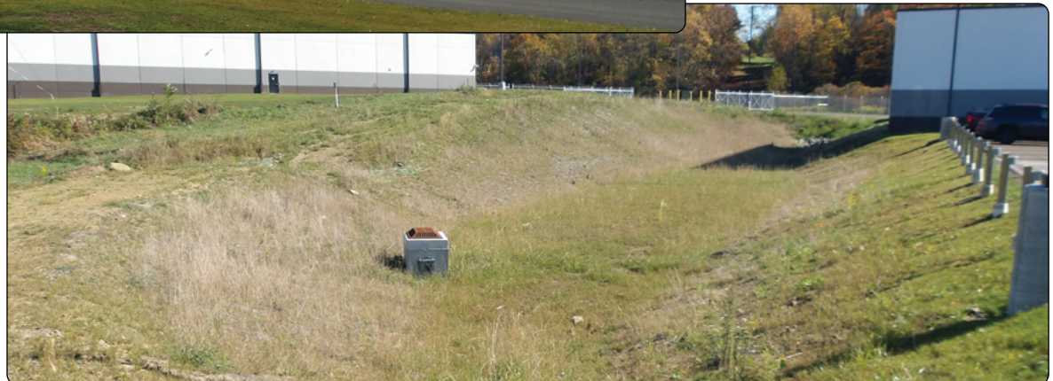
Three stormwater control infiltration basins were installed at the new 300,000 s.f. Fuhrer Eagle Sales & Service warehouse along Route 66 near Delmont.
