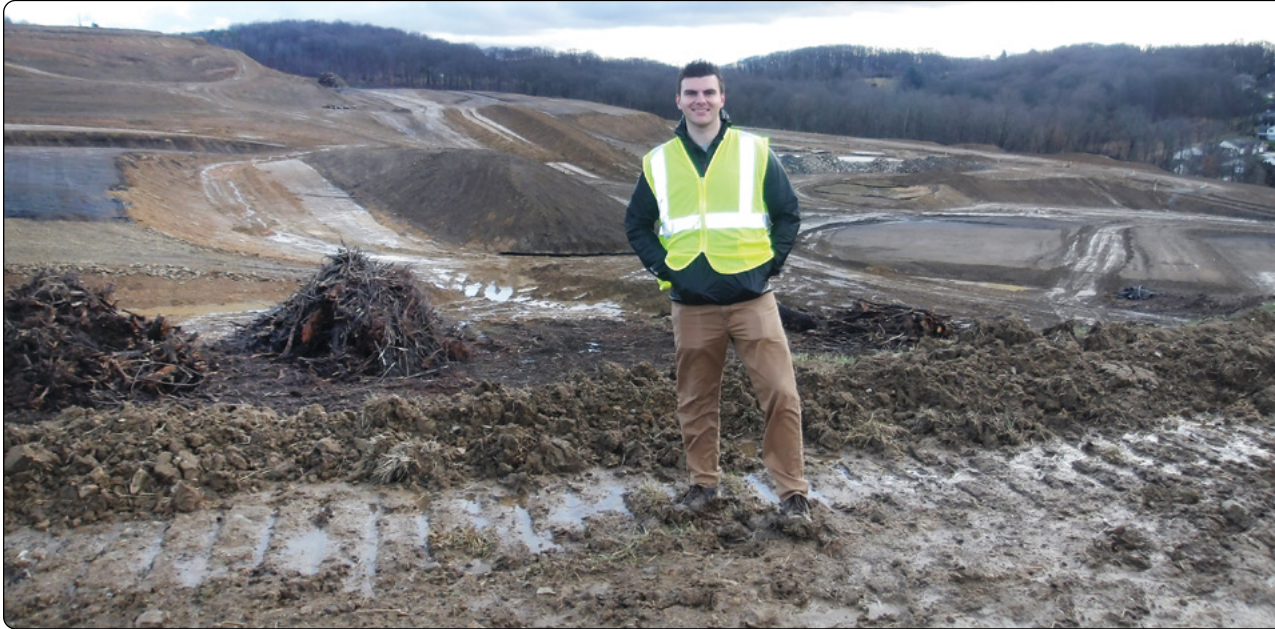
Erosion Control Specialist Ryan Peckheiser inspects the Spyglass Trails residential development site.
