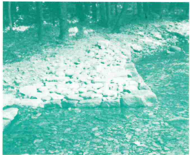
STREAM DEFLECTORS - Located in Linn Run and Jacobs Creek.
