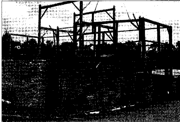
Original frame prior to disassembly...
