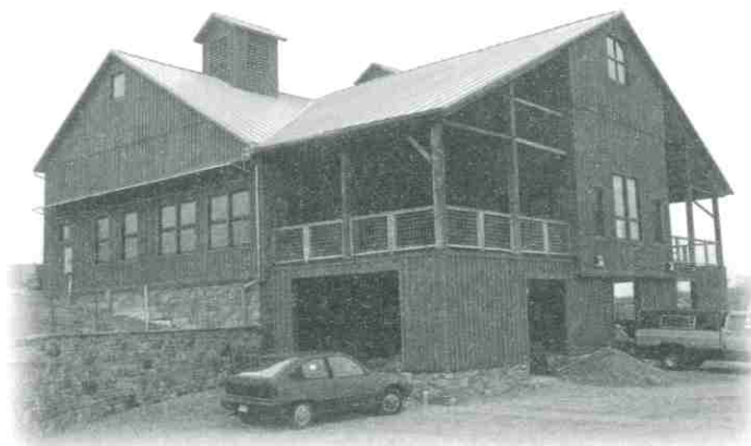
Nestled into the hillside, our Bank Barn shelters office space, meeting rooms, work areas, and even a few field mice!
