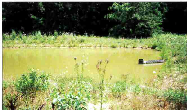
The brown sediment captured by this pond won't end up in a stream.
