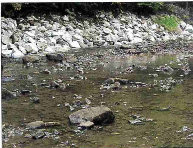
Jacobs Creek near Laurel Run, in Laurelville after stream bank stabilization.
