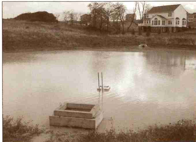
Properly functioning "Faircloth Skimmer" dewater only the cleanest water from the top. This results in 80% sediment removal.
