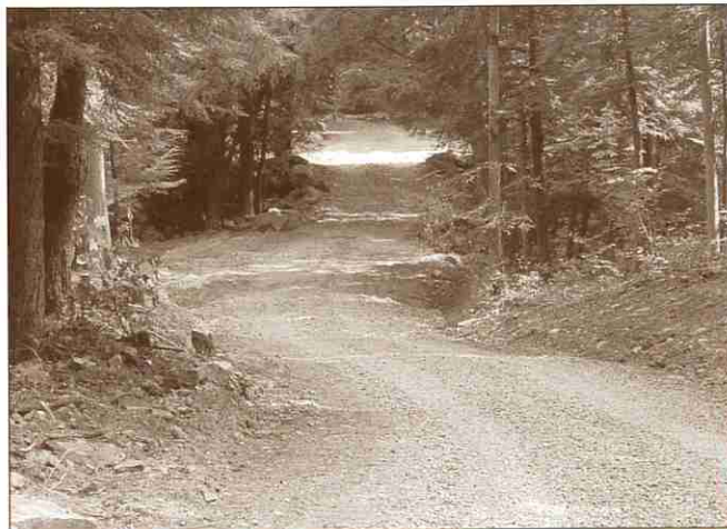
Completed Dirt and Gravel Road in St. Clair Township.
