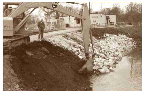
Stabilizing banks of Boyer Run in Sewickley Creek Watershed.
