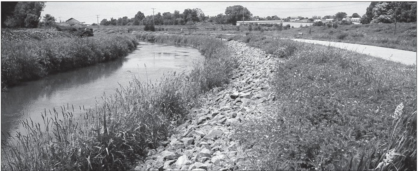
Scottdale Channel. Notice the bank of sediment on the inside bend of the stream (far left), the rock riprap stabilizing the bank on the right, and the hiking/biking trail on the far right.
