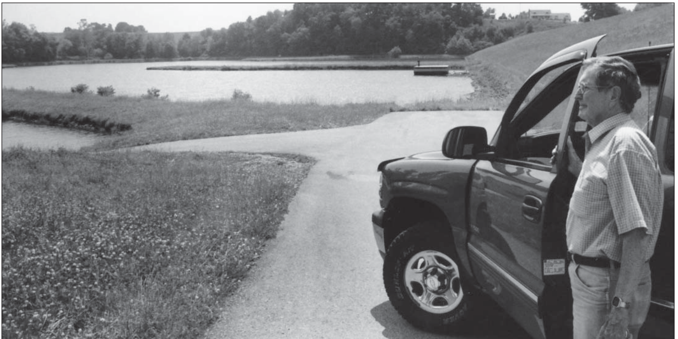
Westmoreland Conservation District Chairman J. Roy Houston stops near the boat launch of the Bridgeport Dam, a flood-control project that maintains a permanent 70-acre water pool for recreation.
