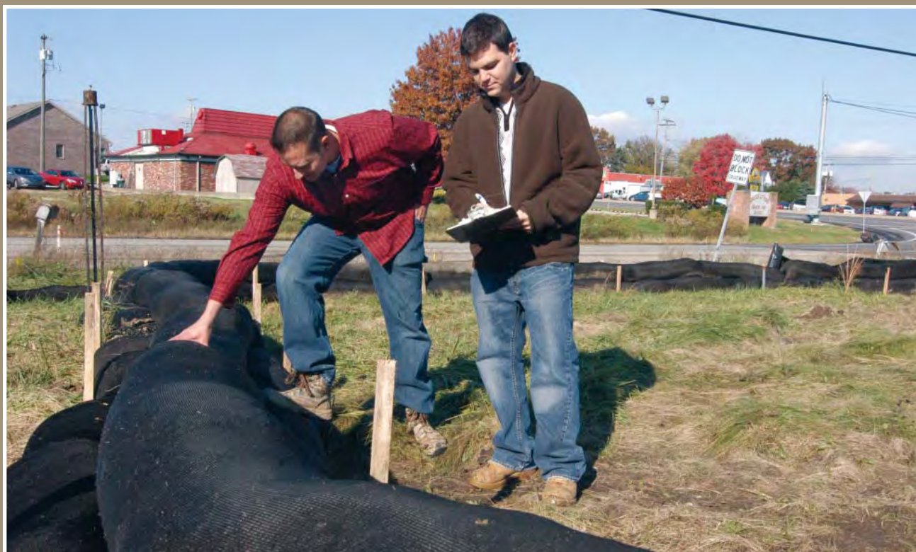
District Senior Erosion Control Specialist Chris Droste (l) and Erosion Control Specialist Matt Zambelli (r) inspect an erosion control barrier at a commercial construction site in Latrobe.
