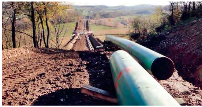
This close up of the natural gas transmission line right-of-way shows its average width of 100 ft.
