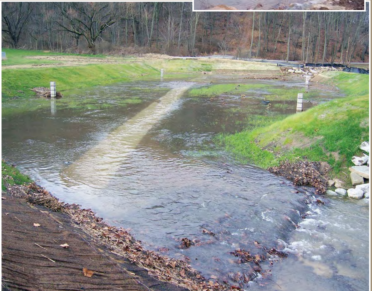
High stream flows are restricted by a row of three-foot square concrete blocks, which direct excess flow and debris into the basin where it is captured. The basin then allows the water velocity to decrease, thus dropping out the debris before the water returns to the creek.
