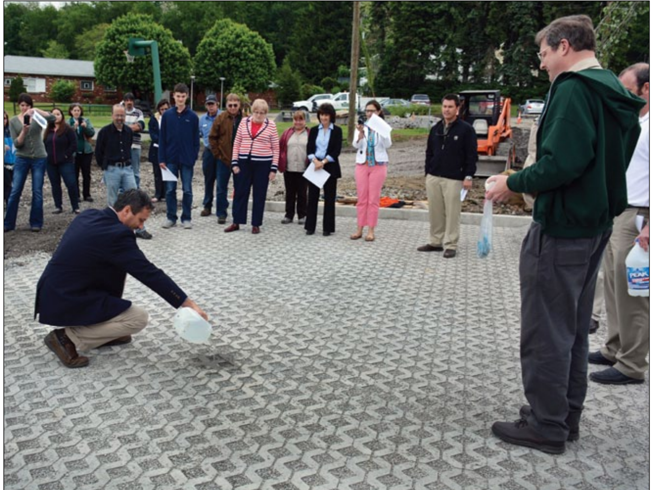
Westmoreland County Commissioner Ted Kopas demonstrates how water easily flows through the new porous parking lot added at the Derry Community Pool in the McGee Run Watershed.
