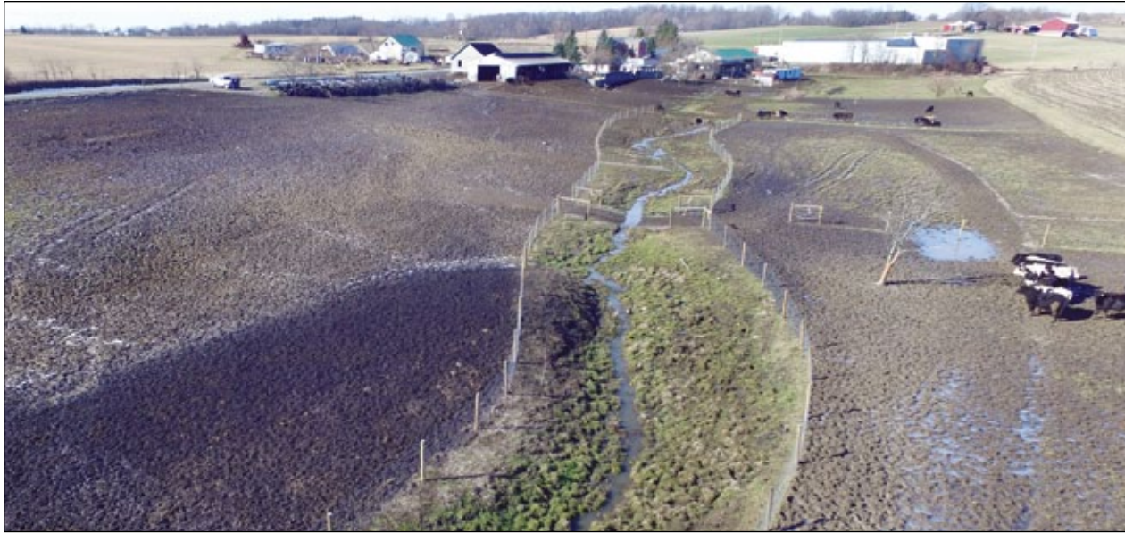
On the Klejka farm in the McGee Run Watershed, some 1,200 feet of fencing was installed along the stream to keep cows out of the water, except at a new limited access crossing area (center of photo), which also was added.
