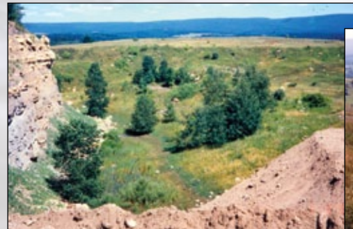
1995 – An 80-foot vertical high wall (foreground) was just one of the many dangerous remnants left behind when coal companies abandoned their mines at the turn of the last century. This site in Ligonier also had steep spoil piles and impoundments of water.
