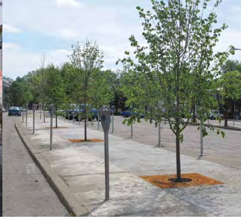
In downtown Vandergrift, a unique underground grid, permeable pavement, and a new row of street trees create a unique and attractive way to manage stormwater.
