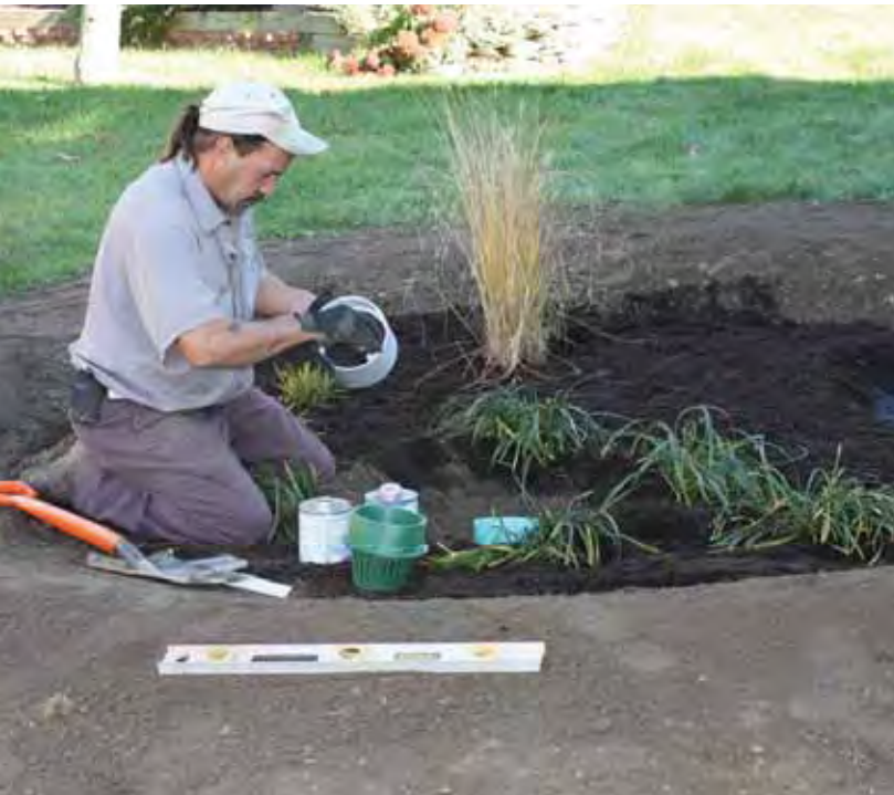
In Mount Pleasant, rain gardens installed in municipal locations and on individual homeowner lots reduce the amount of water flowing into the borough's storm sewer system.
