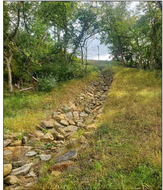
Final rock lined channel
