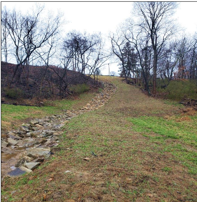
Final channel after stabilization
