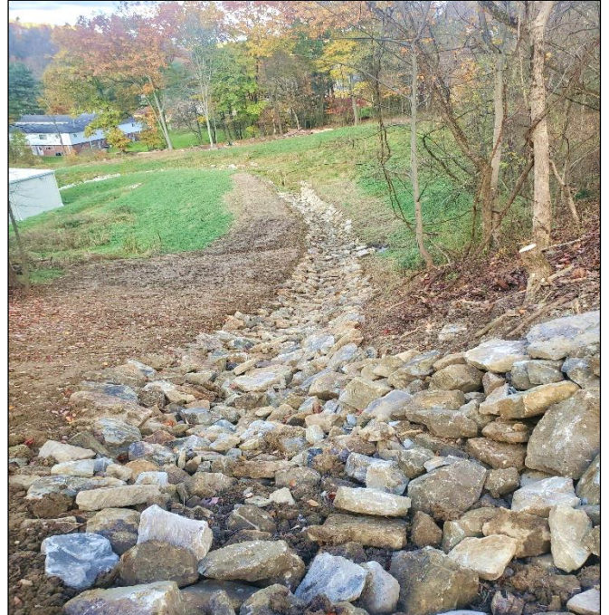
(After) Hillside when channel was under construction and existing channel widened
