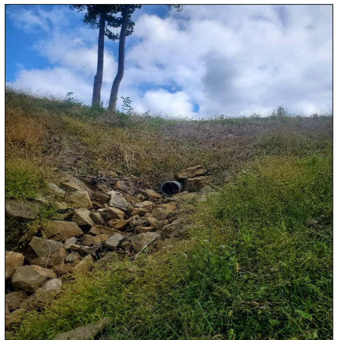
New outlet of pipe and beginning of channel
