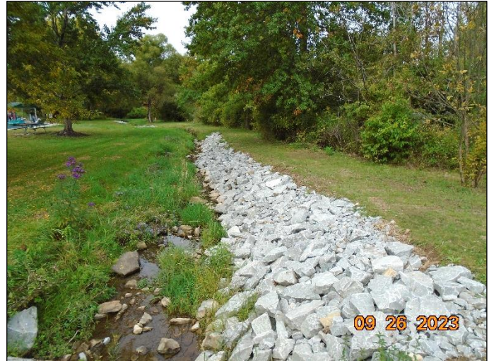
Stabilized streambank by means of bank and dumped rock protection
