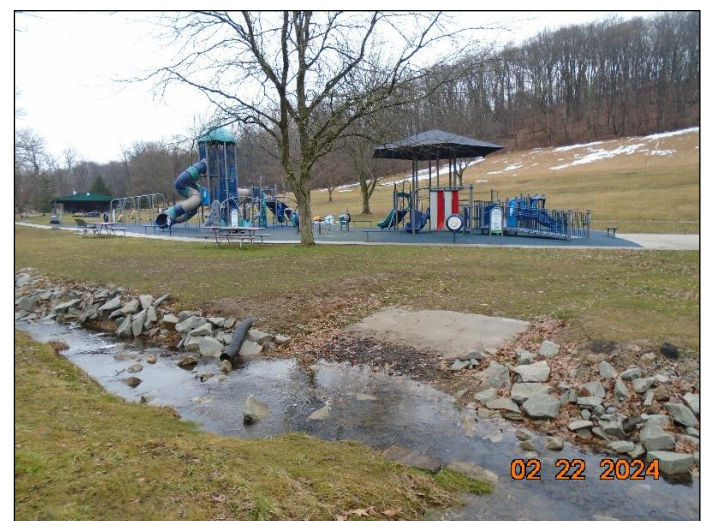
New concrete ramp to allow for educational stream access
