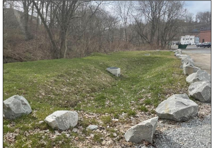
Parking lot retrofitted into two infiltration swales with large rock as natural guide rail.
