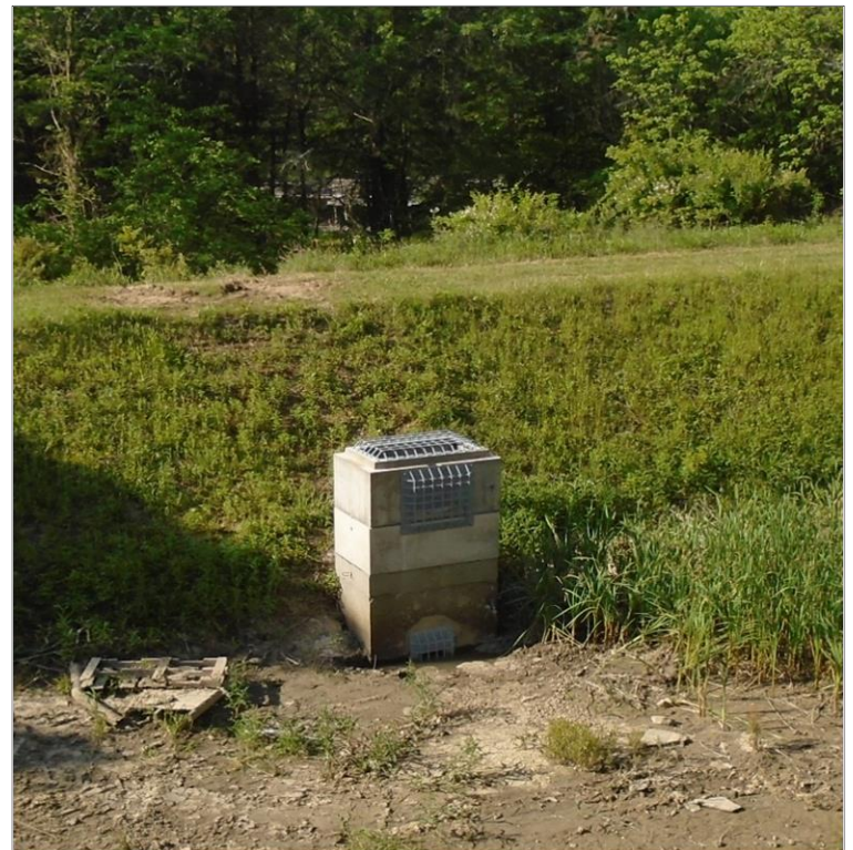
(After) Retrofitted outlet structure with risers and trash racks
