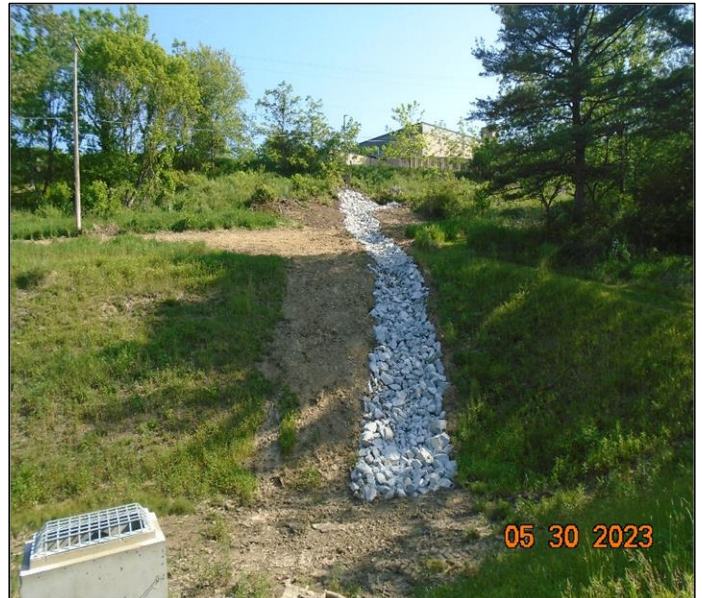
Finished rock-lined channel for stormwater conveyance leading into the stormwater basin
