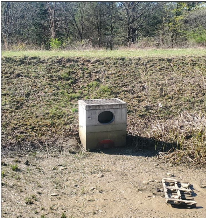
(Before) Stormwater basin outlet structure
