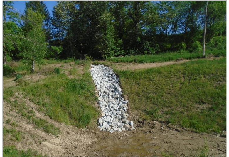
(After) Plastic channel replaced with rock lined channel. Basin restored to original conditions.
