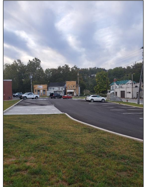
Completed parking lot with permeable parking spots
