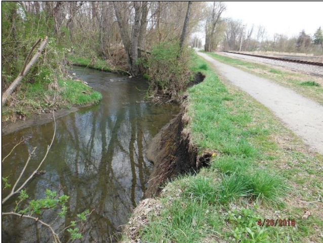
Before: Eroding and vertical banks causing sediment to enter the stream
