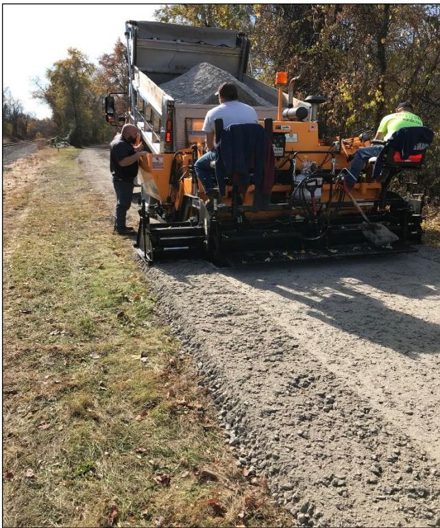
Limestone aggregate paving for trail resurfacing
