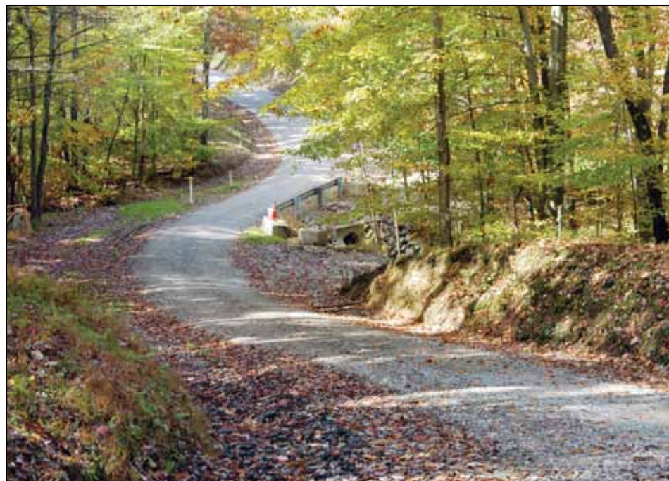
Improvements to Larimer Trail Road in Washington Township will not only make travelling easier for motorists but, by reducing erosion, will keep more than 40 tons of sediment out of waterways in the Kiskiminetis Watershed each year.
