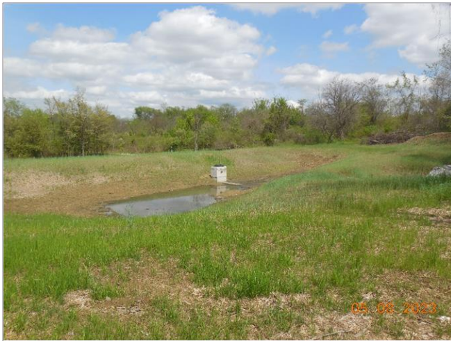
(Before) Stormwater basin after construction
