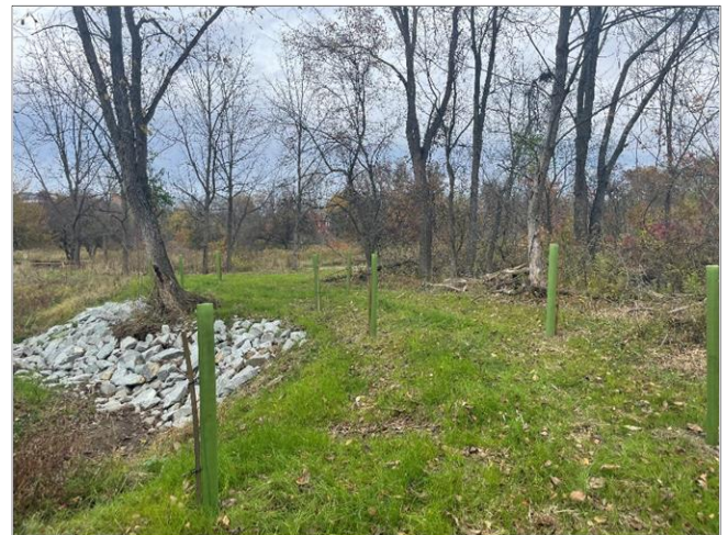
Native tree plantings that were installed to assist with stream bank stabilization and riparian buffer development
