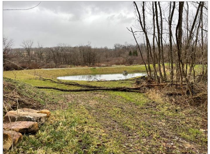
Stormwater basin with limestone surface trail and educational sign
