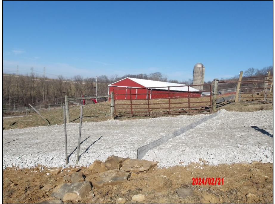
Stabilized Animal Walkway with Conveyor Belt Diversions.
