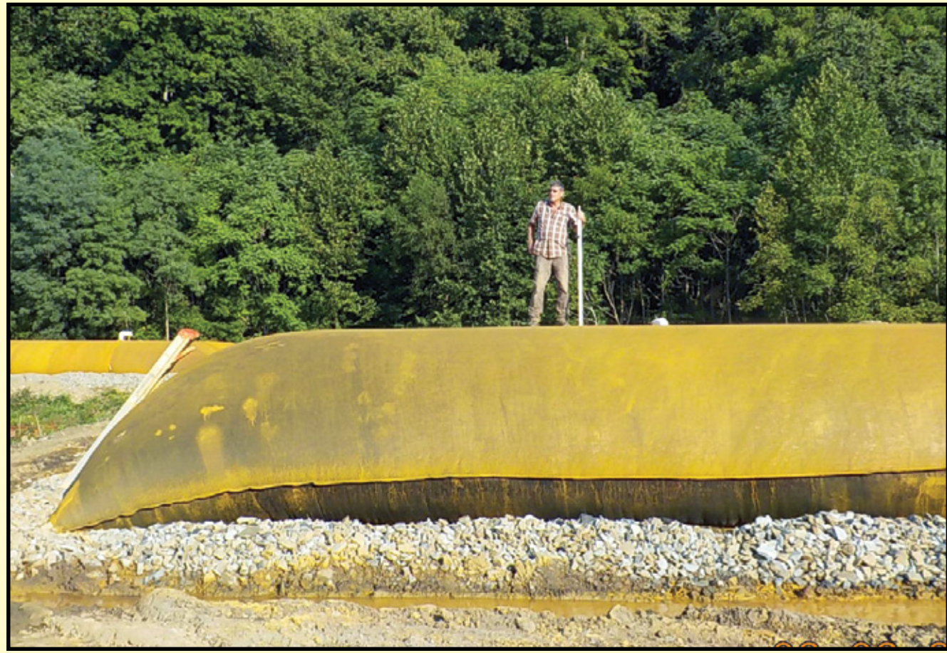
left: Iron oxide is regularly harvested from the bottoms of the ponds, then dried and sold for commercial use. right: A large geotube (drying bag)
