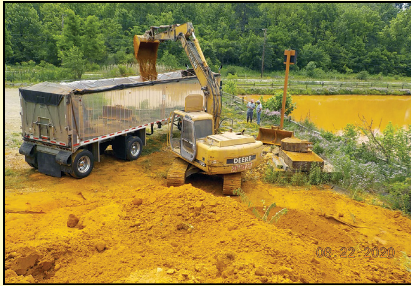
left: Iron oxide is regularly harvested from the bottoms of the ponds, then dried and sold for commercial use. right: A large geotube (drying bag)
