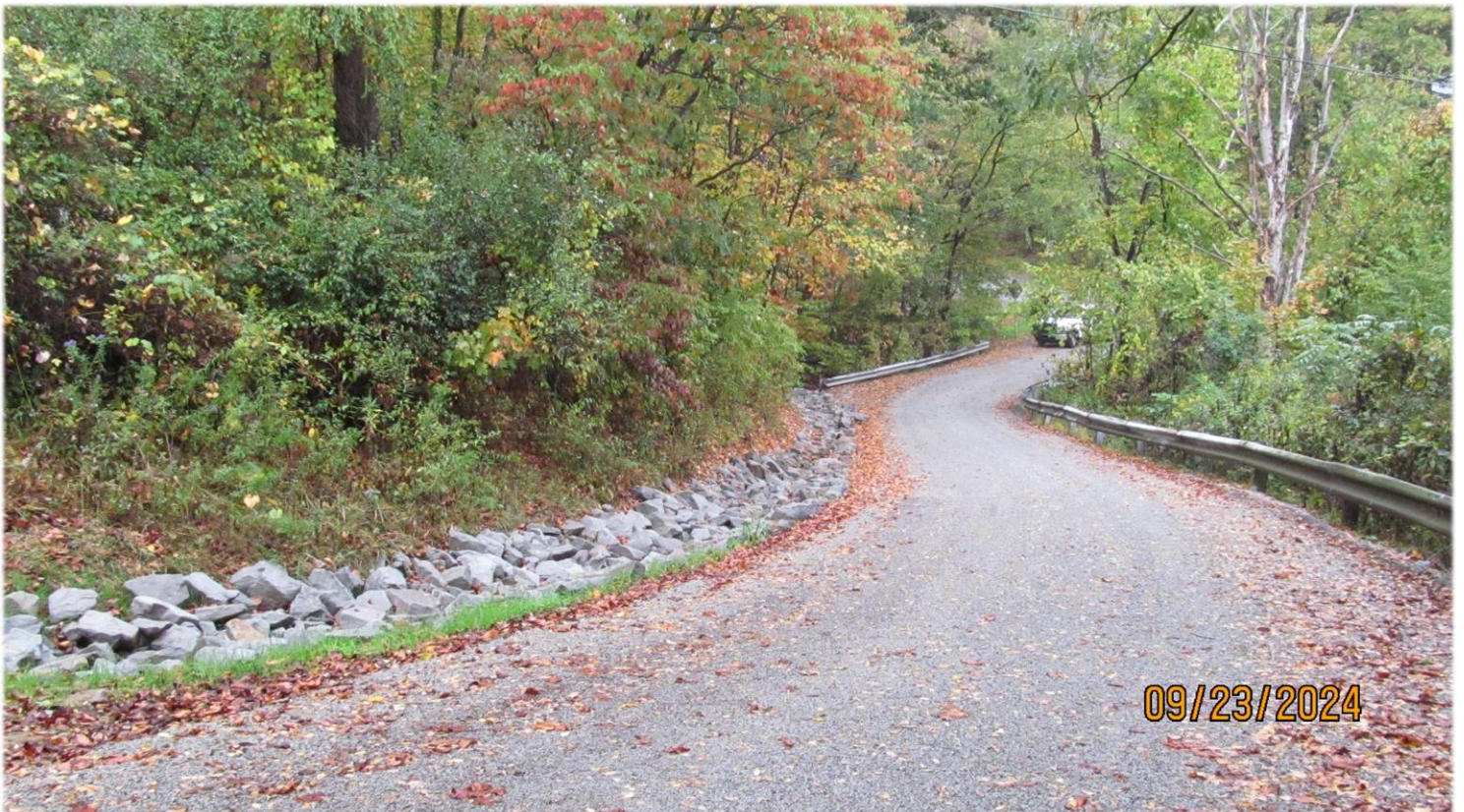
(After): Stabilized ditch line and stabilized surface
