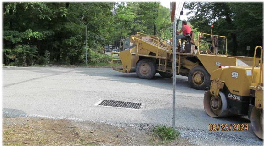
Road surface being sealed with tar and chip
