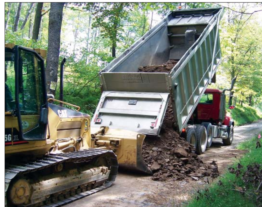
The addition of pipes for drainage (left) and raising and stabilizing the road surface (right) have made Larimer Trail Road better for drivers and the nearby stream.
