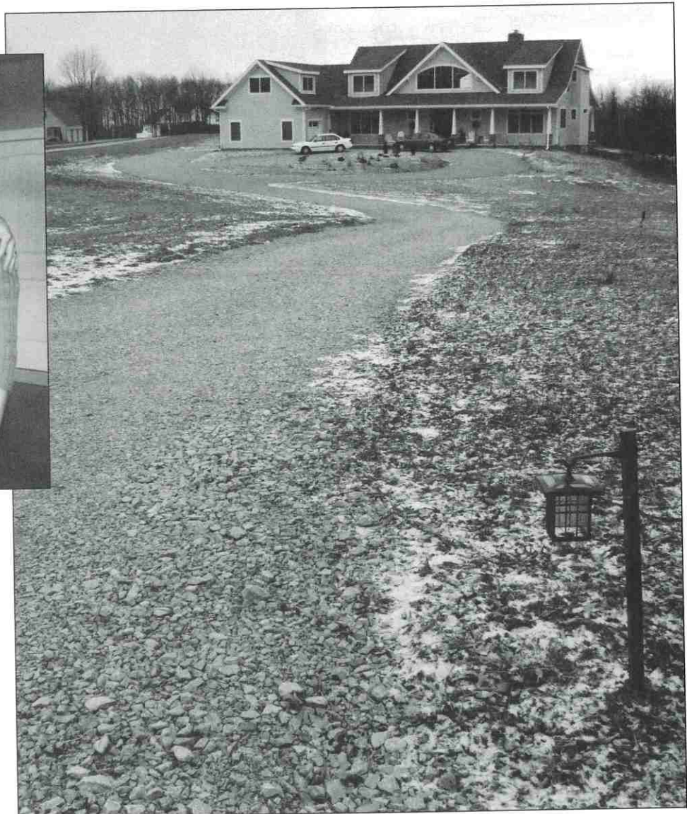
After learning about the importance of infiltrating stormwater, the Grants decided not to pave their 300-foot driveway, but to keep it in gravel.
