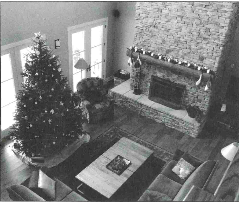
Large low-E windows, a simulated stone fireplace, and a mantel made of a 300-year-old wormy red oak log from a cabin in Bullskin Township reflect the family's conservation ethic and bring elements of nature and history into the home.
