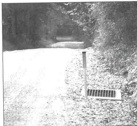
New catch basin installed along Lupyan Road in Loyalhanna Township.
