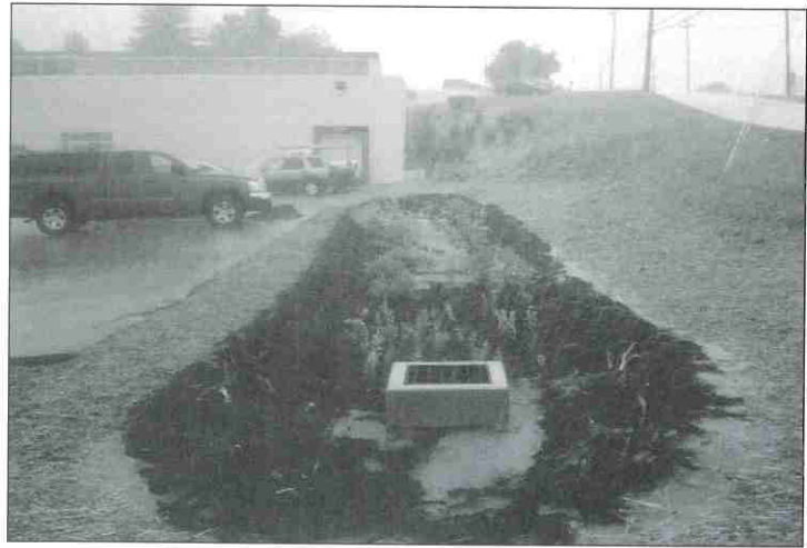
New swale for GreenForge building.
