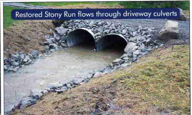
Restoring the streambed
