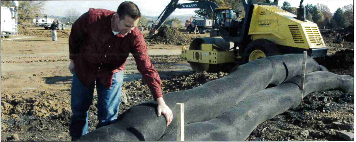
Barriers help keep loose soil from migrating off construction sites.
