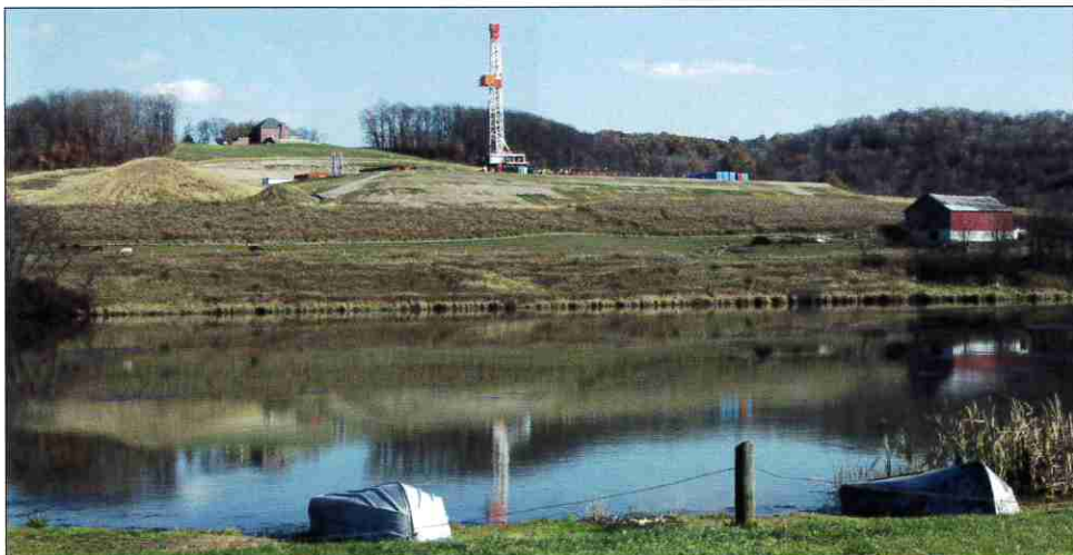
Gas well near Donegal Lake, just off Route 711, in Donegal Township.
