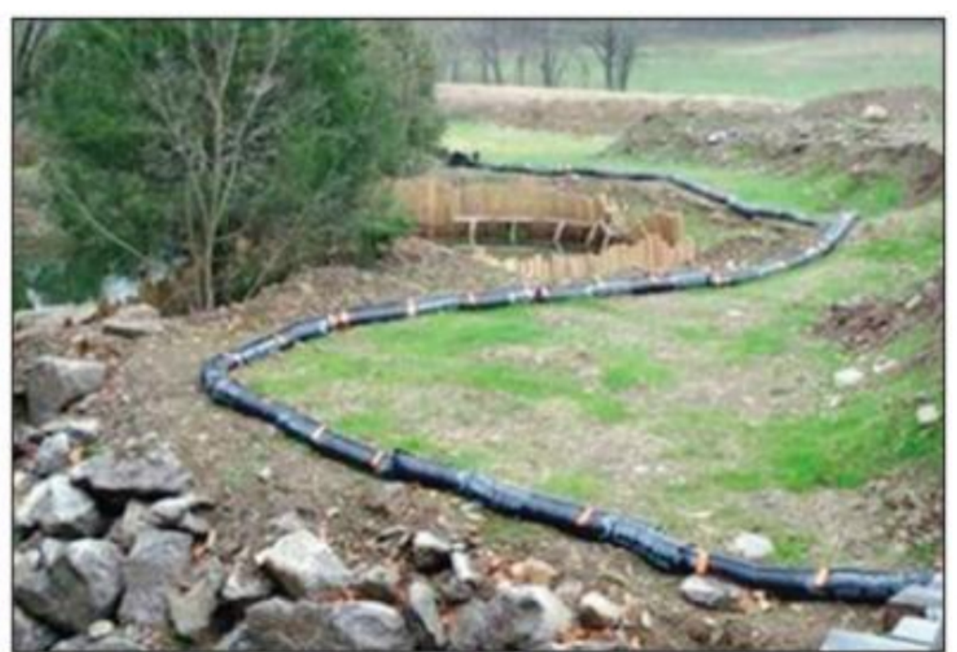
Filter tubes are aligned end to end to control runoff.
