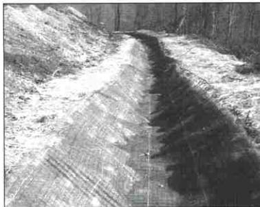
(left) This giant collector ditch gathers sediment and takes it to a collection basin/trap for sediment removal before discharge to the stream.
