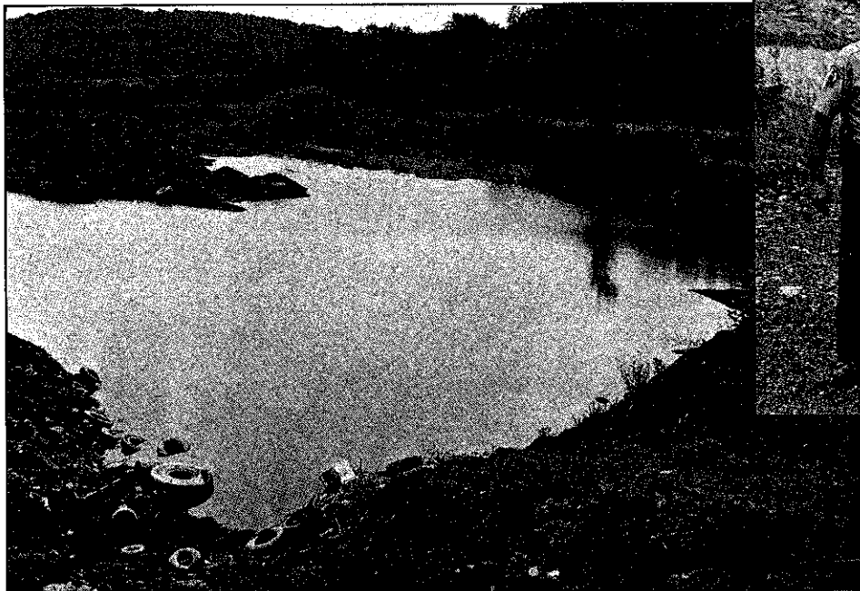
Impounded water and trash, abandoned mine site, Washington County, PA
