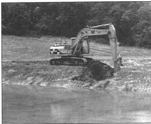
Working on wetland #3.
