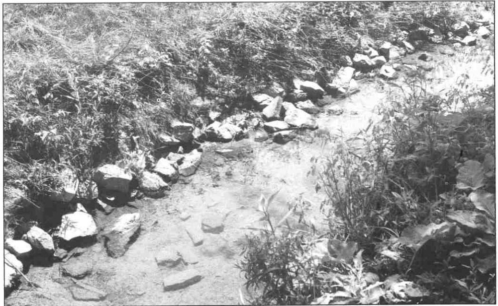
The stabilized streambank, Lynch Field, Greensburg.
