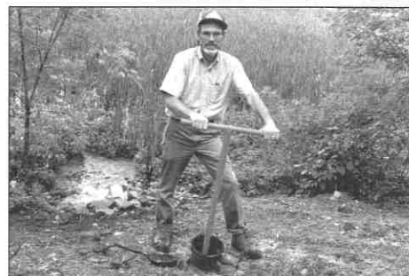
Helping design and build the passive AMD wetland treatment system at Saint Vincent College.
