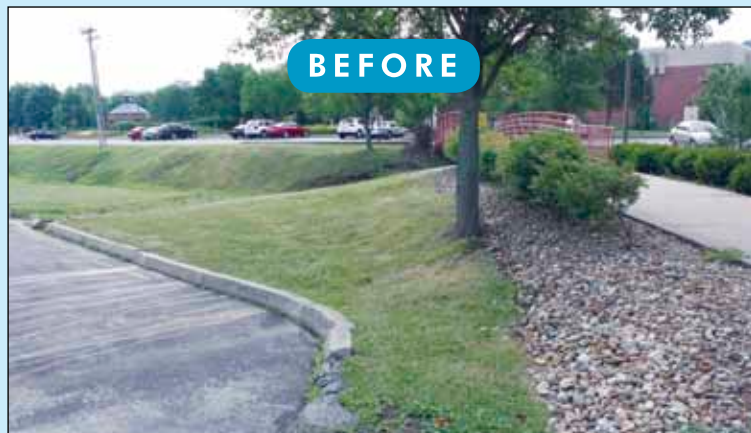
Asphalt dominated the landscape near the creek increasing the volume and velocity of stormwater runoff from the parking lot.
