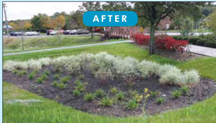
Here's the same view. The asphalt was replaced by a rain garden, which will absorb stormwater to nourish its attractive plants and shrubs.
