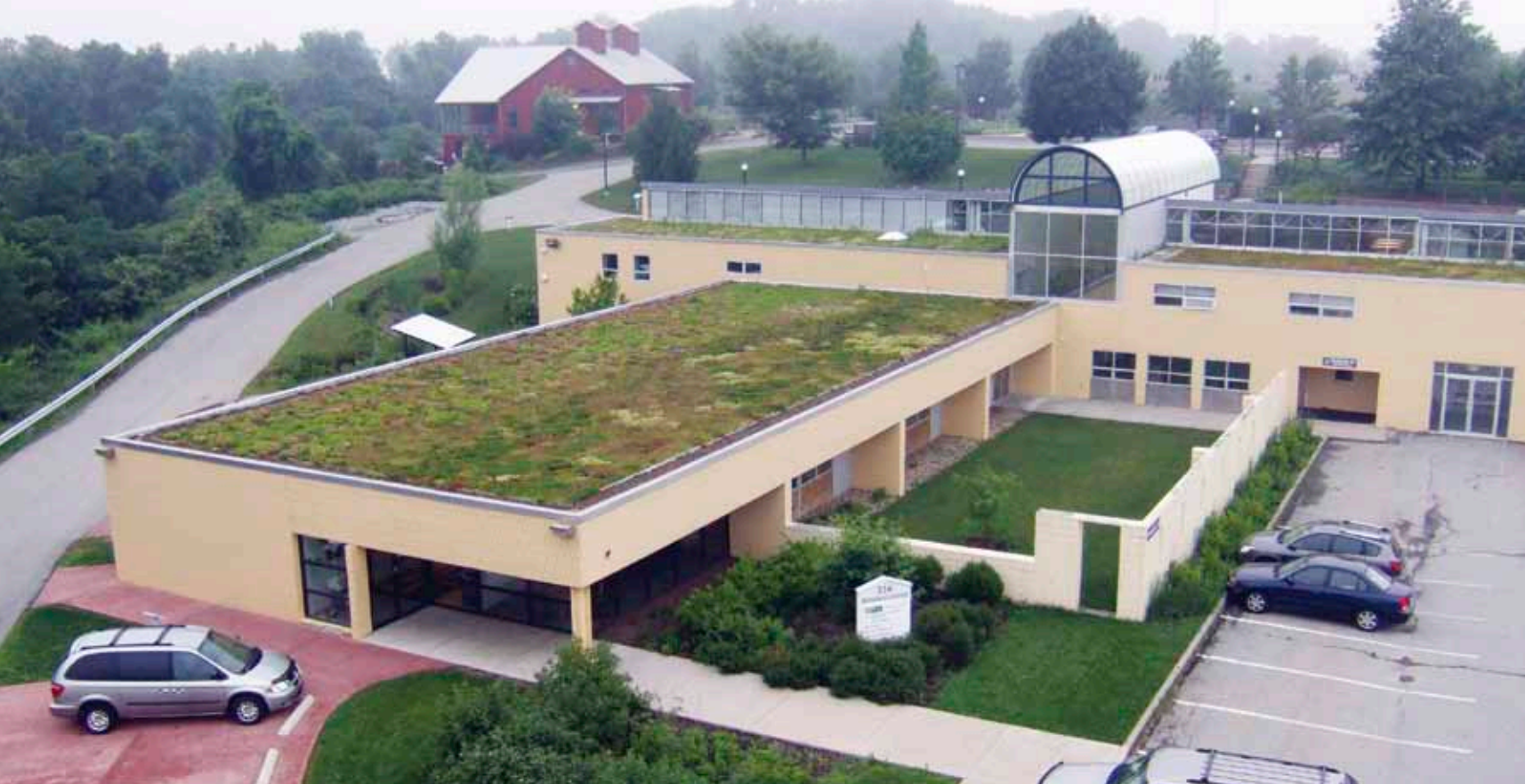
A view of the GreenForge building's green roof with the Conservation District barn in the background on the Donohoe Center Campus
