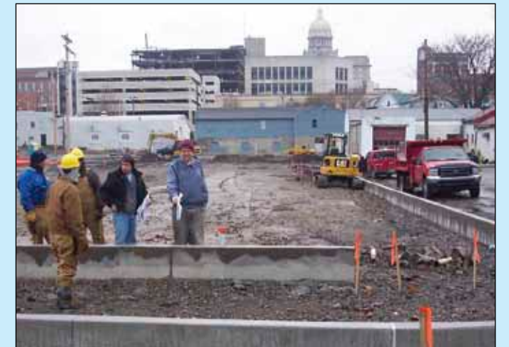
Construction begins on the Moore Avenue lot.
