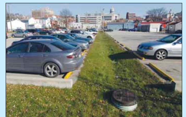
Stormwater runoff infiltrates into the ground from the grass swales.
