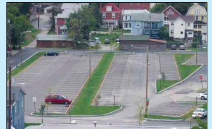
Grass swales between the rows of parking collect runoff.
