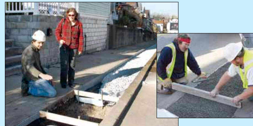
left photo (l-r), Jarod Trunzo, Community Engagement and Sustainability Coordinator for the City of Latrobe and Kathy Hamilton, RLA, District Stormwater Technician, discuss the placement of street trees along Lloyd Avenue. right photo: Workers smooth out porous concrete, which will help nourish the street trees when it rains and reduce maintenance for residents. For more photos visit us on Facebook.
