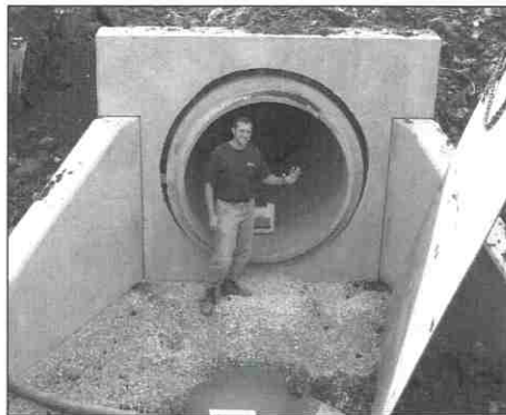
Chris Droste, WCD inspector standing in the 5 foot Diameter Stormwater collection pipe headwall near the Koelsch Property
