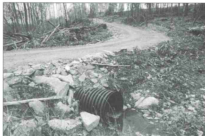
This photo shows how the harvesters properly used a "Best Management Practice" (pipe and stone) to build the haul road across a stream.
