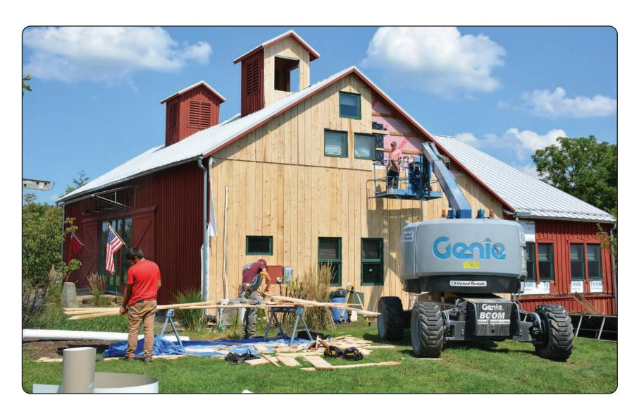
The District barn received a major upgrade to the exterior with new siding of local hemlock, high quality structural sheathing panel, and a moisture control barrier
