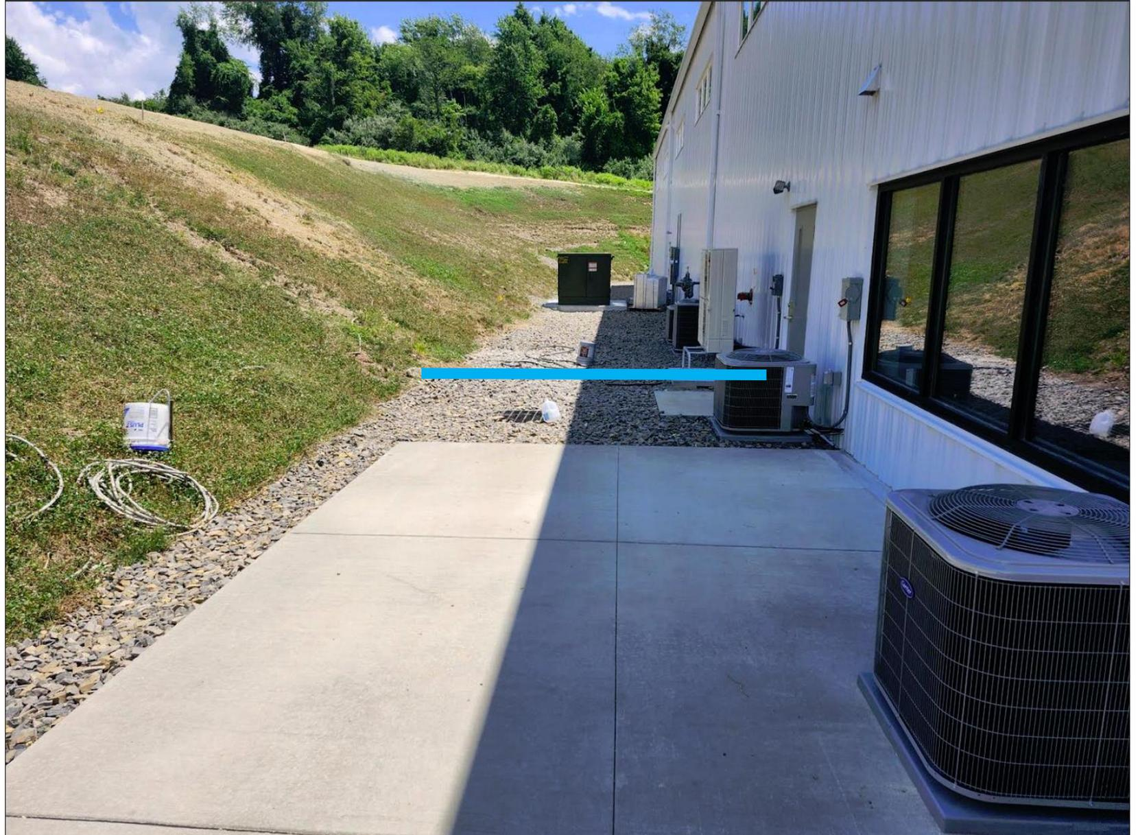
This rock-lined ditch is not really a ditch at all. Without capacity inside the ditch, water will start running alongside the ditch outside of the rock.
