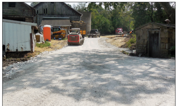
Stabilized access road was installed to grant better access to the milkhouse, barns, and concrete liquid manure storage.
