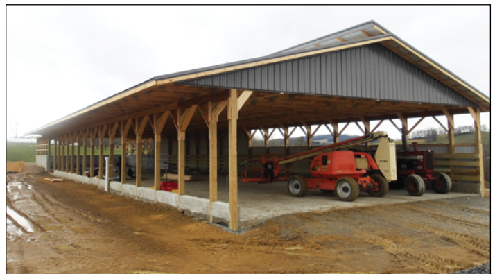
C. McChesney Farm roofed animal heavy use area with a manure staking pad installed to house beef cattle.
