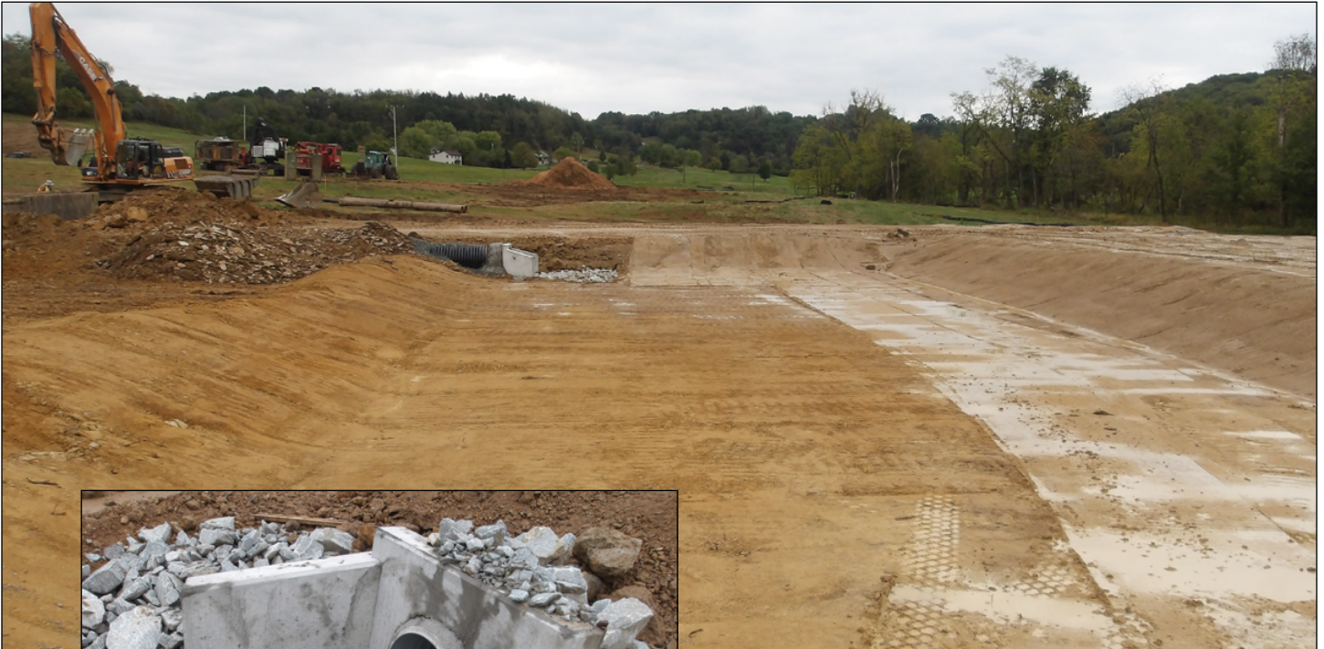
Above: The first sediment basin constructed at Valley Green Estates used to catch sediment laden water from the construction site.
