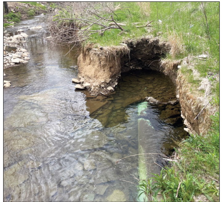
Eroded streambank and exposed sanitary sewer line in Washington Township.
