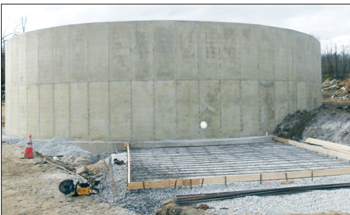
A concrete liquid manure storage tank and agitation prep pad.
