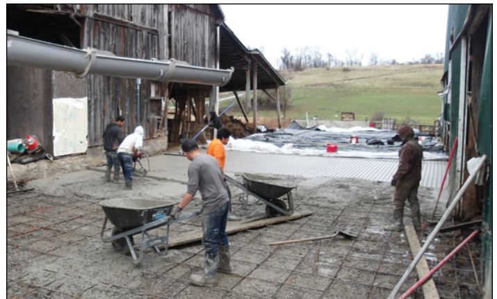
New concrete being poured to create a stabilized pad between the barns.
