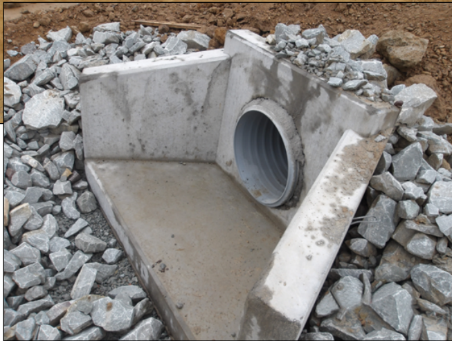
Above: The first sediment basin constructed at Valley Green Estates used to catch sediment laden water from the construction site.
