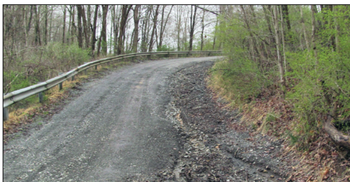
Before: Unstable gravel surface and eroding ditches.
