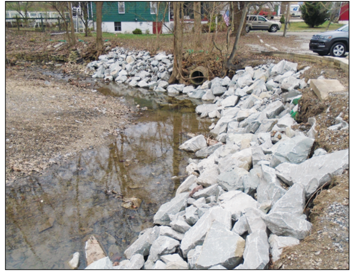
After: The streambank area was stabilized with riprap.
