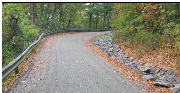
After: Stabilized surface and ditch line.
