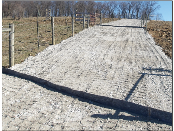
After: Stabilized animal walkway with three conveyor belt diversions.
