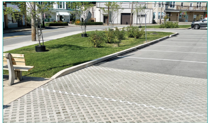
The Foundation recently helped rehabilitate this parking lot in Manor Borough with rain gardens, trees, shrubs and permeable pavement to help control stormwater and add greenspace.
