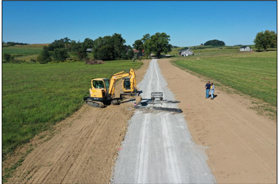
Stabilized Animal Walkway with Conveyor Belt Diversion Installation
