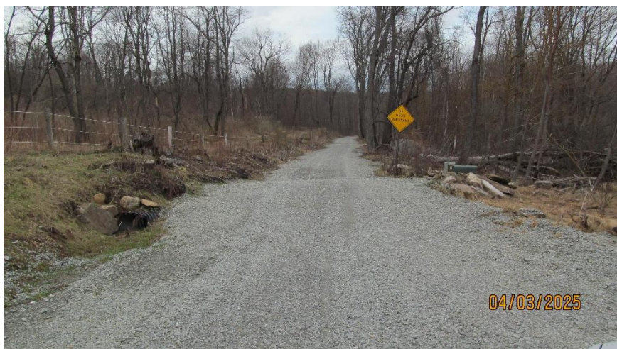
(After) Road built up with gravel and grade breaks to divert the flow of water and stabilize driving surface.
