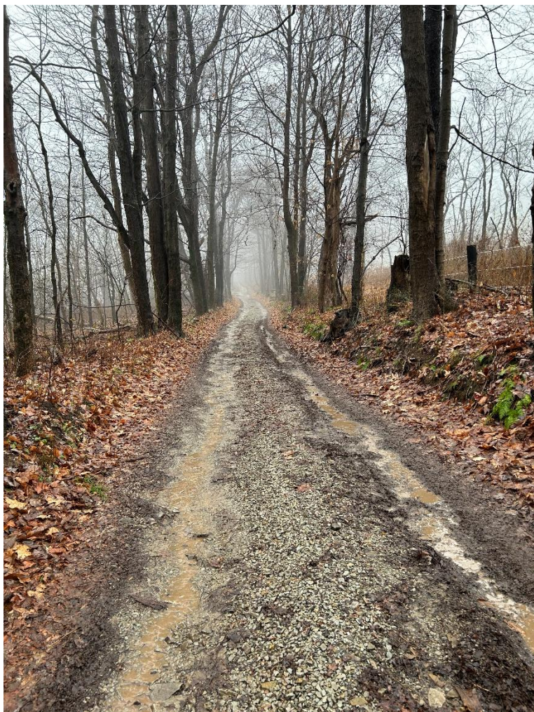
(After) Road built up with gravel and grade breaks to divert the flow of water and stabilize driving surface.
