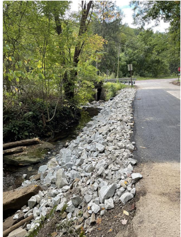
Finished streambank stabilization showing the stabilized roadside.
