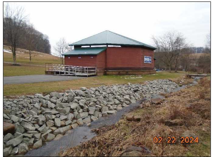
Streambank stabilization by means of bank grading and dumped rock protection
