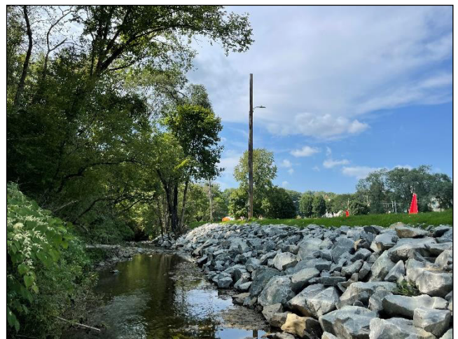
(After) Banks graded back to a stable slope and rock added to the toe of the slope.
