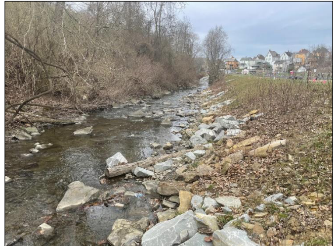
(After) Banks graded back to a stable slope and single log vane deflectors (10) installed to stabilize eroding streambank.
