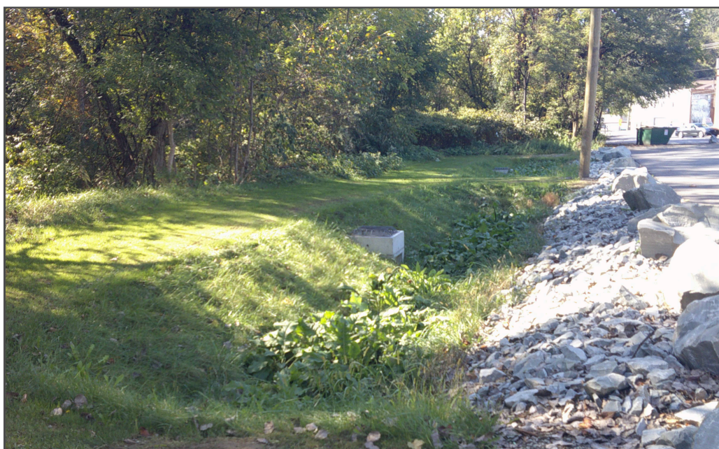
Infiltration swale two years after construction
