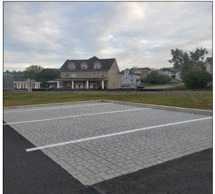
Eco-optiloc permeable pavers
