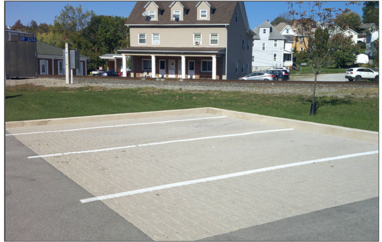
Premeable pavers two years after construction
