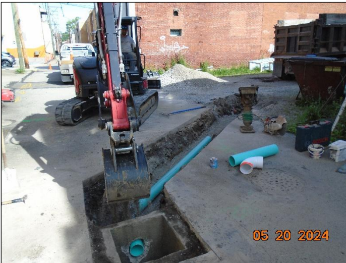
Pipe connection from the rain garden to an existing inlet
