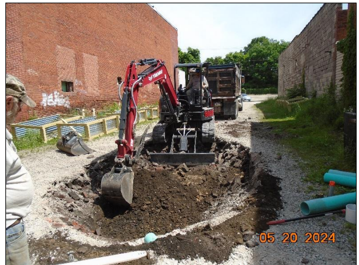
Excavation of the rain garden
