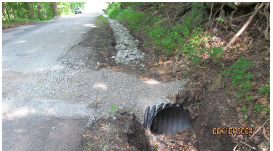
(After) Cross pipe added from one side of the road to the other.
