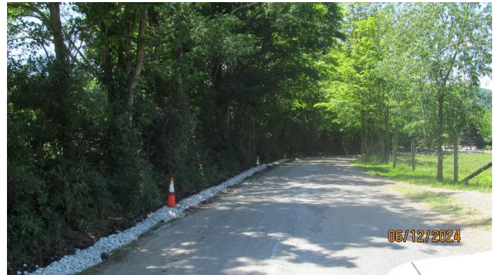
Filling the ditches of the road with stone.
