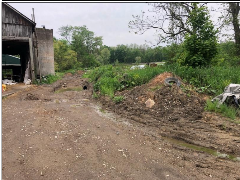
Before: Eroded farm access road.
