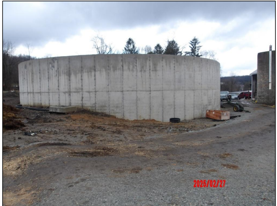
Installed liquid manure storage
