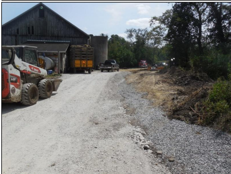
After: Farm access road stabilized with stone and subsurface drainage installed.
