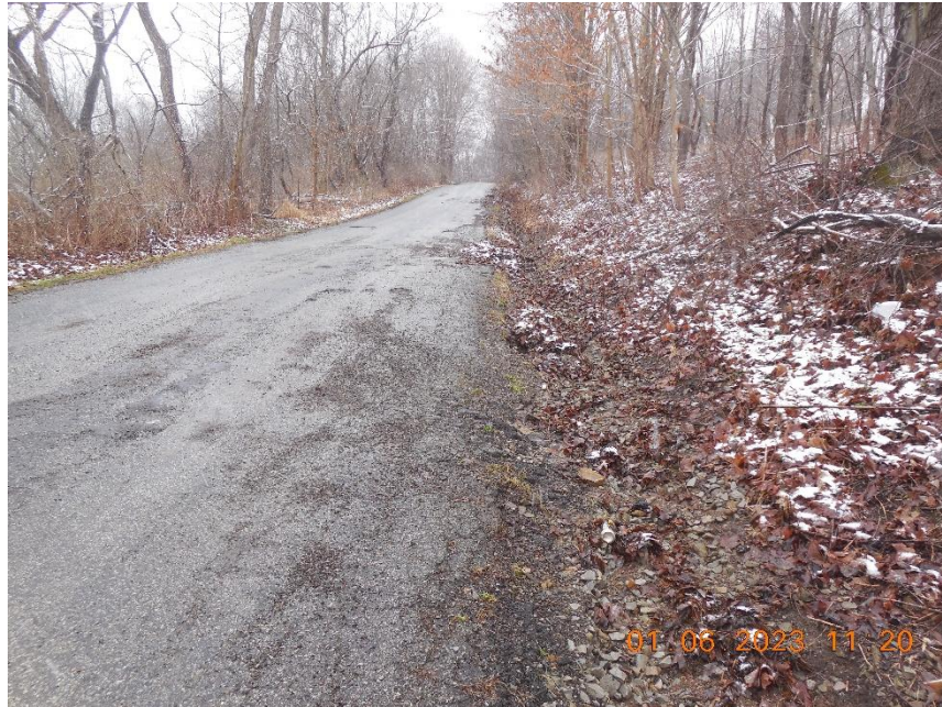
(Before) Sediment building up on the side of the road before underdrain with gravel was added.
