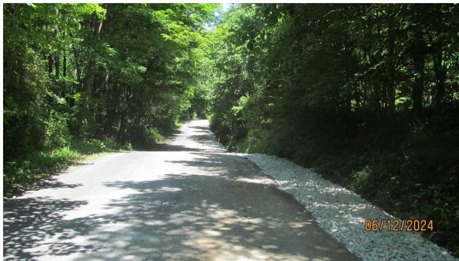
(After) Underdrain on the side of the road with gravel overtop to reduce sediment pollution and flooding.
