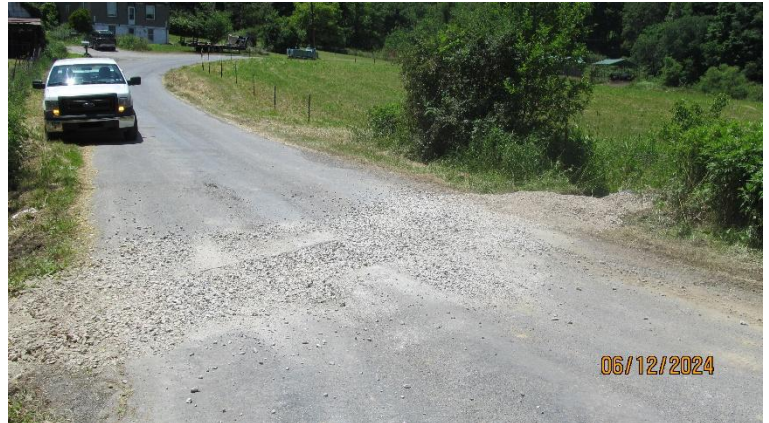
Newly added cross pipe to convey water from one side of the road to the other.
