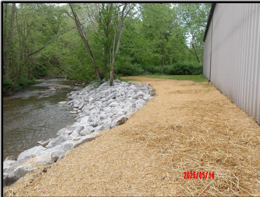
After: Stabilized streambank and yard area restored.
