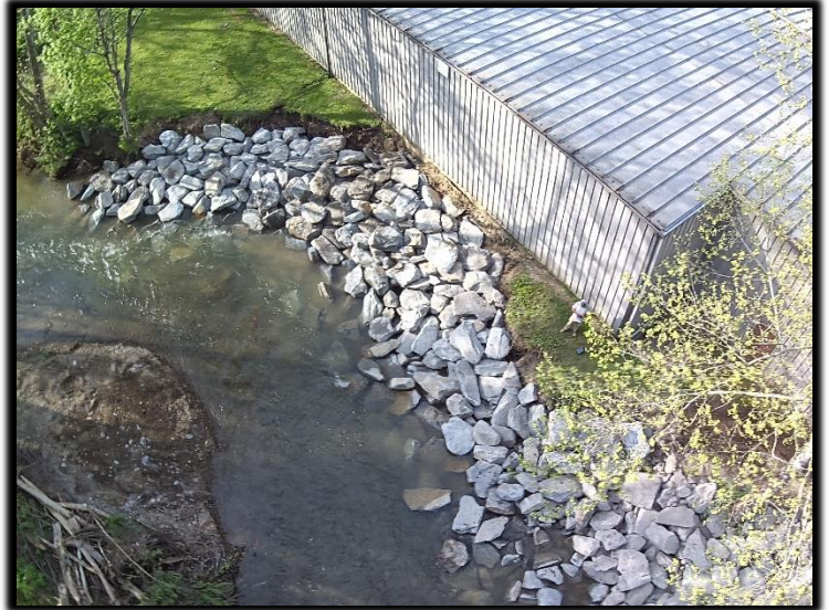
During: Large R-8 size rip-rap installed to restore eroding streambank.
