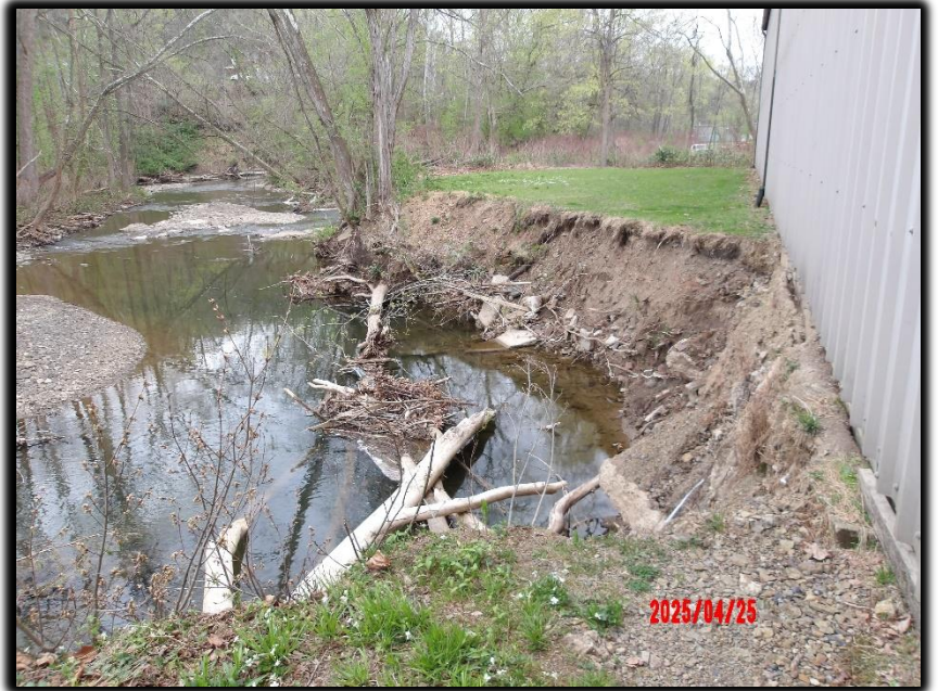
Severe streambank erosion threatening the back of the Style-Rite Kitchens building.
